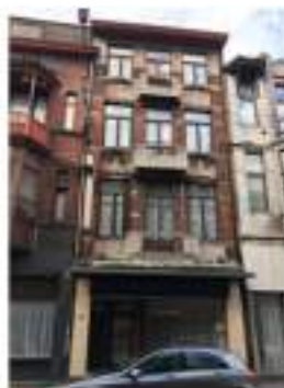
C. Need of maintenance
